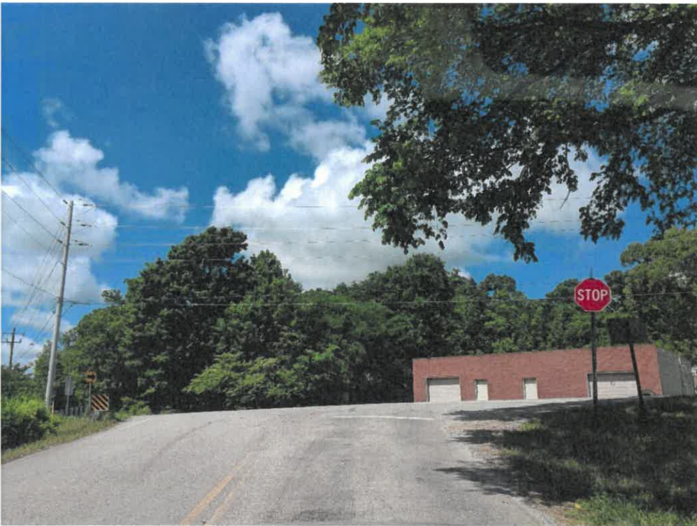
Project terminus on Unitia Road. Photographer facing southwest.
